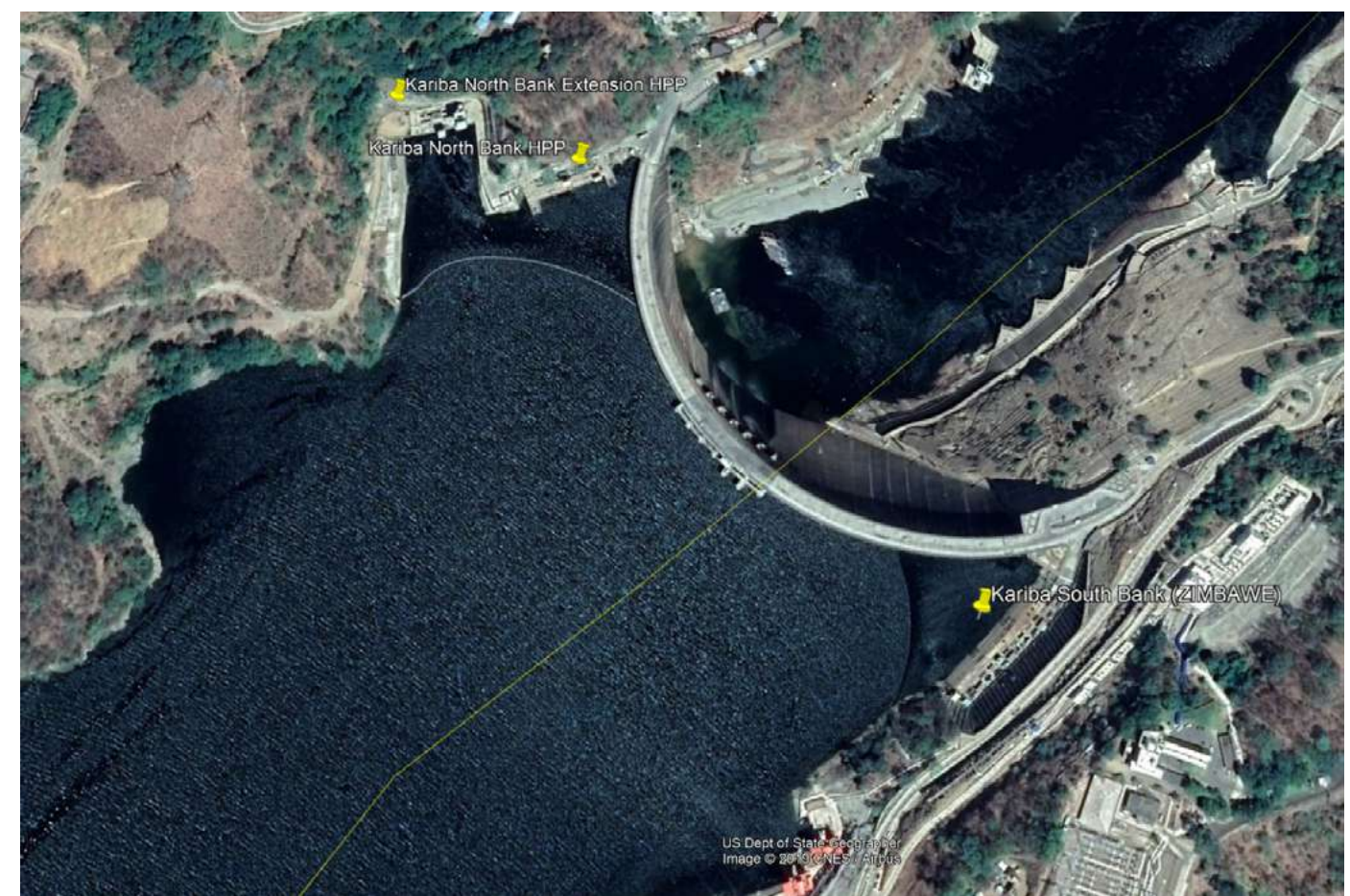
Figure 6.31 – Existing power plants at Kariba lake dam
